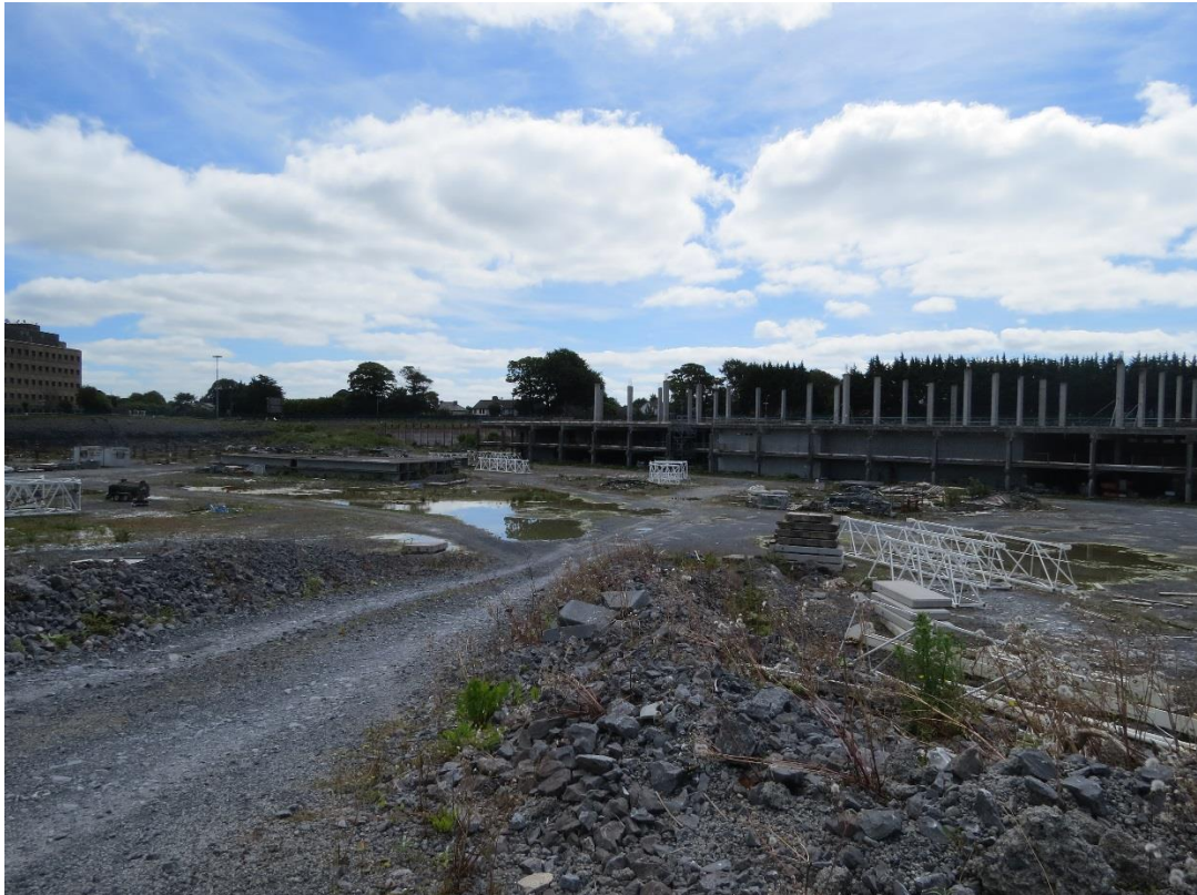
Image 1: Existing construction on site (abandoned in 2008)
