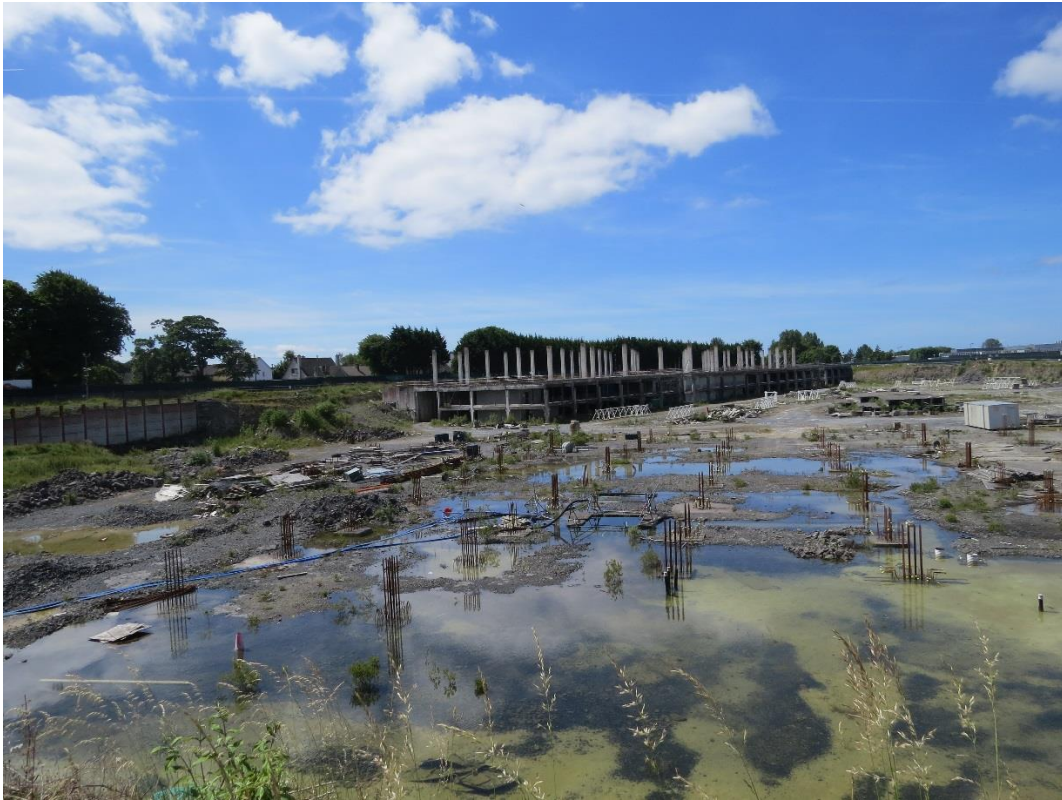
Image 5: Ponding water on existing foundations
