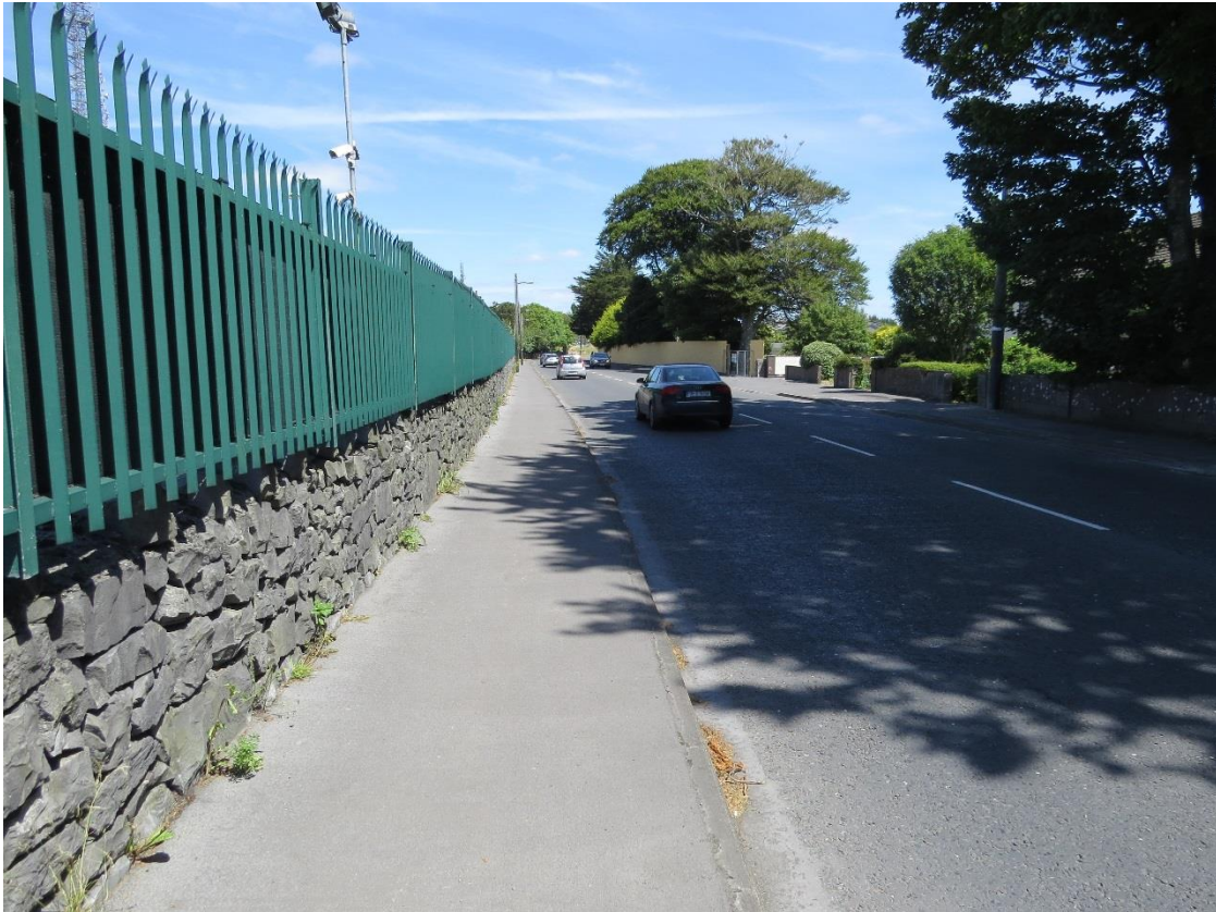
Stage 7: Stone wall with railings on South side of site.
